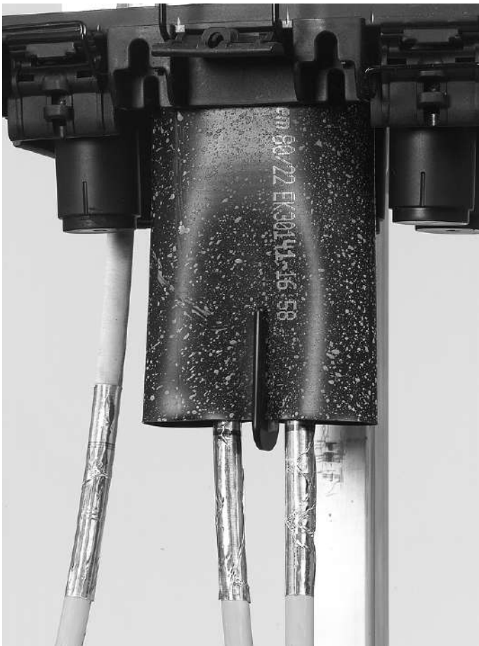
8.2.1.4. Push the sleeve against the base and install the clip.
