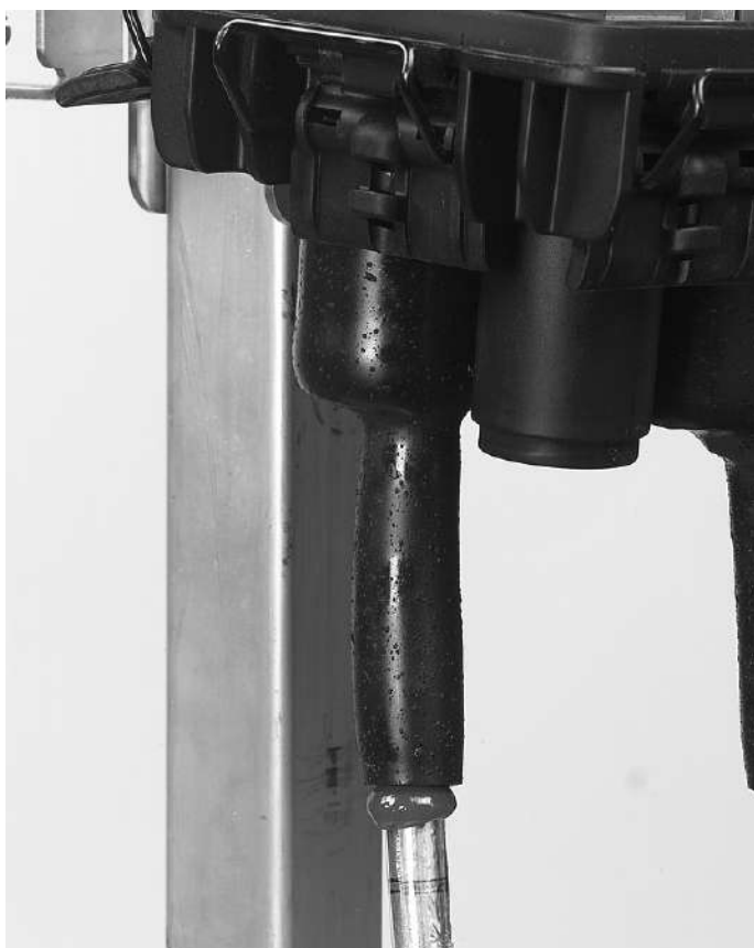
8.2.2.4. Drop cable sleeve installed.
