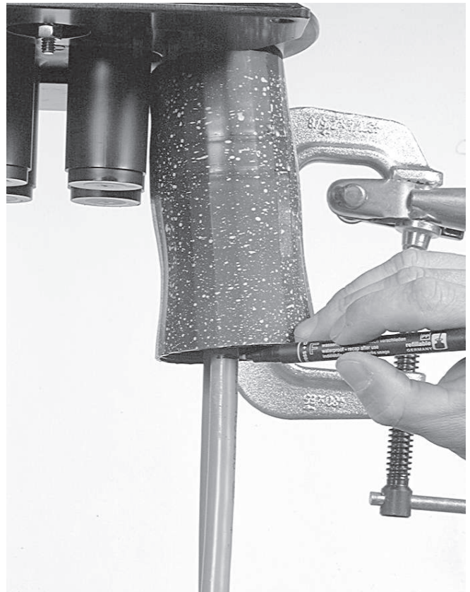
5.1.3 Remove the packing bag out of the sleeve, push the sleeve upwards to the base and mark the cable flush with the sleeve. Make sure the non-coated zone butts up against the base.
