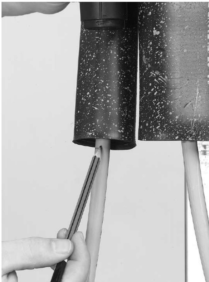
8.2.2.3. Mark the cable with the end of the sleeve. Make sure the sleeve butts up against the base.
